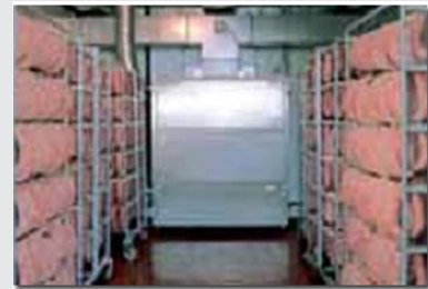
Cold Storage Room
